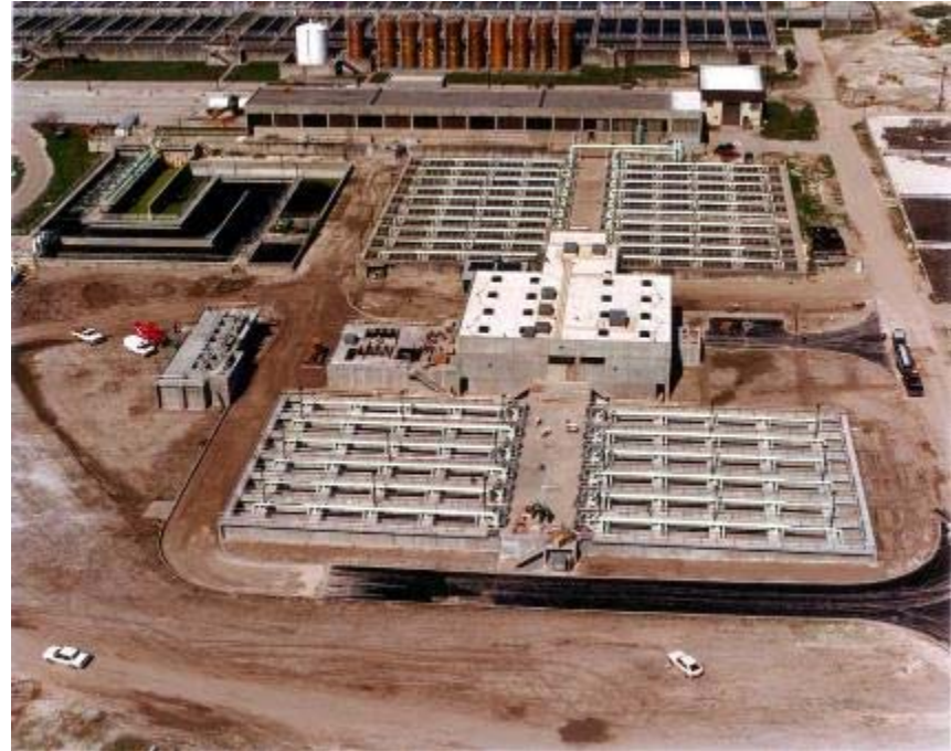
Howard J. Curran WWTP Tampa, FL Denite Filters with 100 MGD capacity
